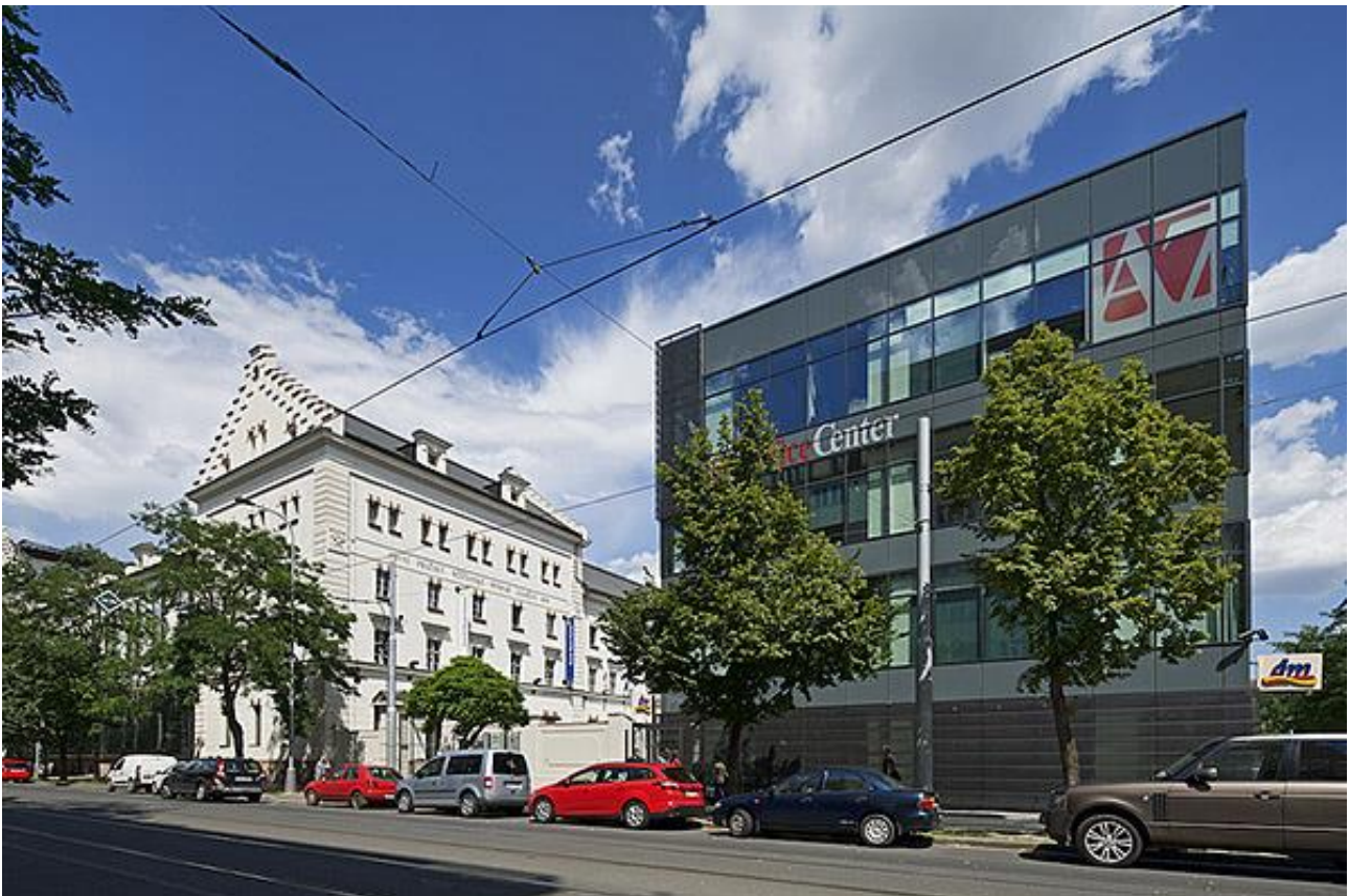
A7 Office Center, Prague (Czech Republic)
